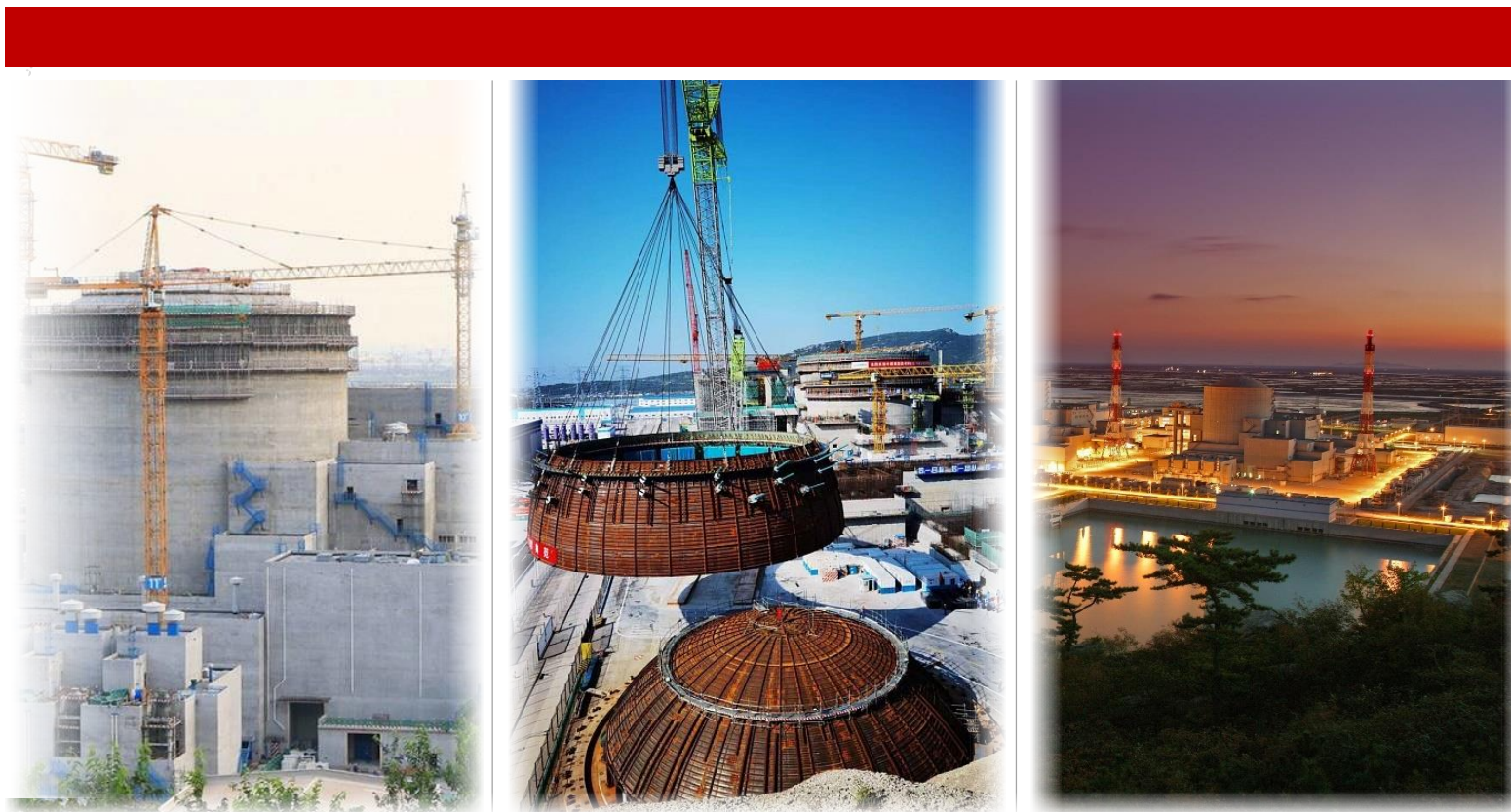
Construction of the Tianwan and Xudapu NPPs in China
